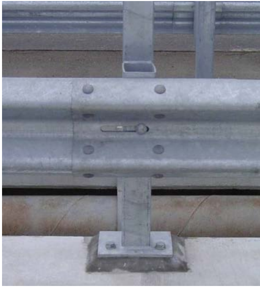
Figure 1 Bridge W-Beam Guardrail (3.4mm thick) (150mm long post bolt slot)
