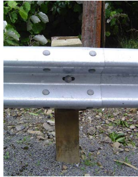
Figure 2 Highway W-Beam Guardrail (2.7mm thick) (63mm long post bolt slot)
