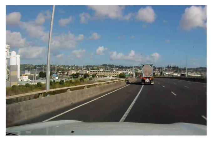
**Issue**: Standard light pole access panel is not on road side. In this case this means a cherry picker is required for inspections, creating a fall from height and working over water hazard.
