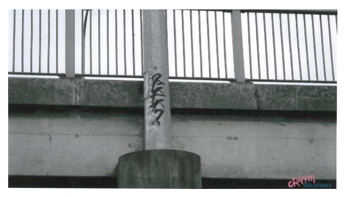
**Issue**: Light pole plinth design creates an easy access point for graffiti vandals. To clean the graffiti, a motorway lane closure is required to establish a safe work platform (e.g. scissor lift).
