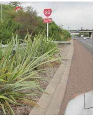
**Issue**: Poorly located vegetation around barriers requires maintenance to prevent it becoming a road safety hazard. This leads to shoulder closures and a less safe workplace.
