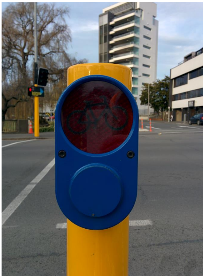
Figure M01 – Cycle call accept indicator (no call present). * Note – Blanking plate fitted to push button as automatic detection installed.
