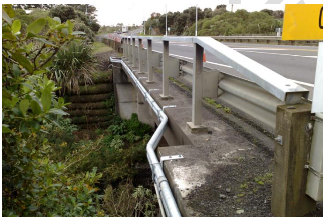
Figure 5. Typical galvanised steel ducting on the side of a bridge.
