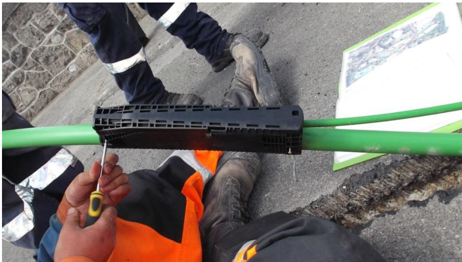
Figure 10. Example of a commercial (green) direct-buried ducting connector being installed. These connectors allow a spur to be broken out of the duct line. The spur itself is broken out from the backbone fibre at an upstream joint. The spur fibre is thus blown from joint to asset through this connector. This enclosure is directly buried into the trench (visible on the right). These are green ultra-fast broadband ducts.
