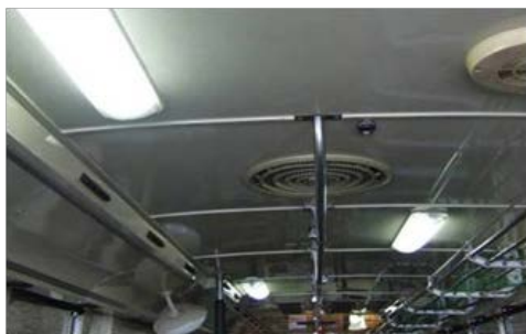
Adequately illuminated interior lighting.
