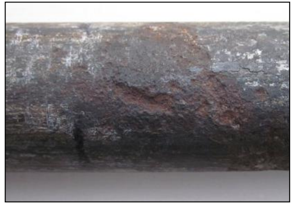
Figure 52. Corroded area on 38.1 mm diameter linkage bars recovered from Kaiapoi Railway River Bridge.
