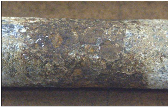
Figure 51. Corroded area on 25.4 mm diameter Linkage bars recovered from the Ahuriri River Bridge.
