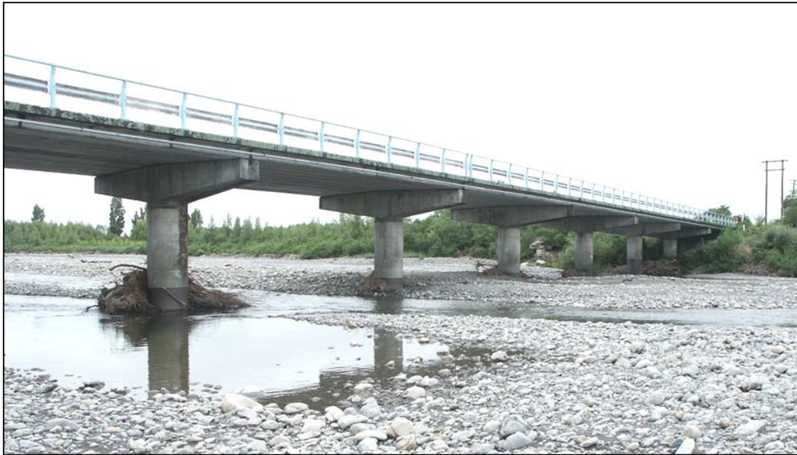
Figure 55. Tauherenikau River Bridge looking towards the east end.
