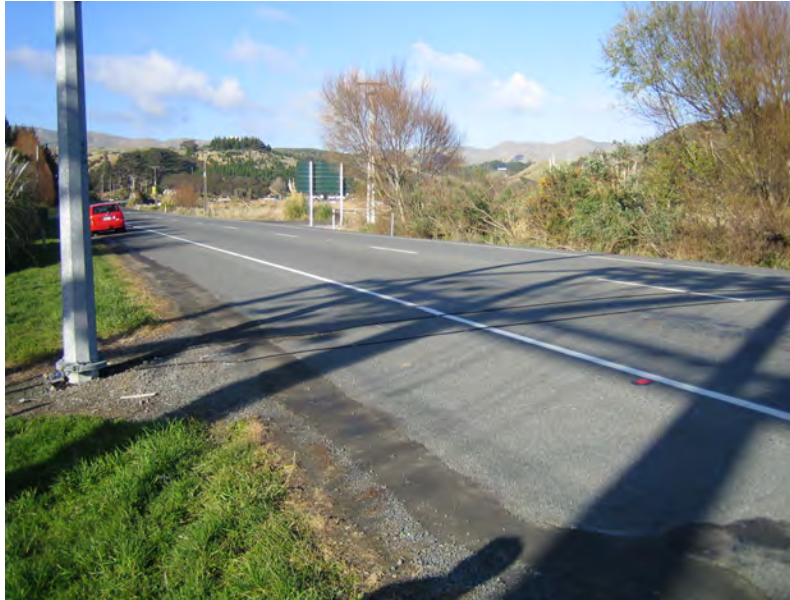
Figure 3: Vehicle classifier installation for Site 6e, downstream location 12
