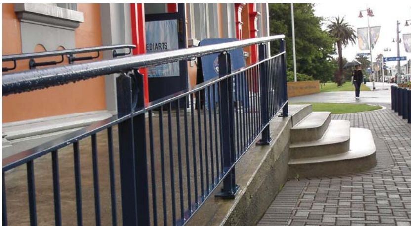
Photo 16.5 – Pedestrian fence, Hamilton (Photo: Shane Turner)
