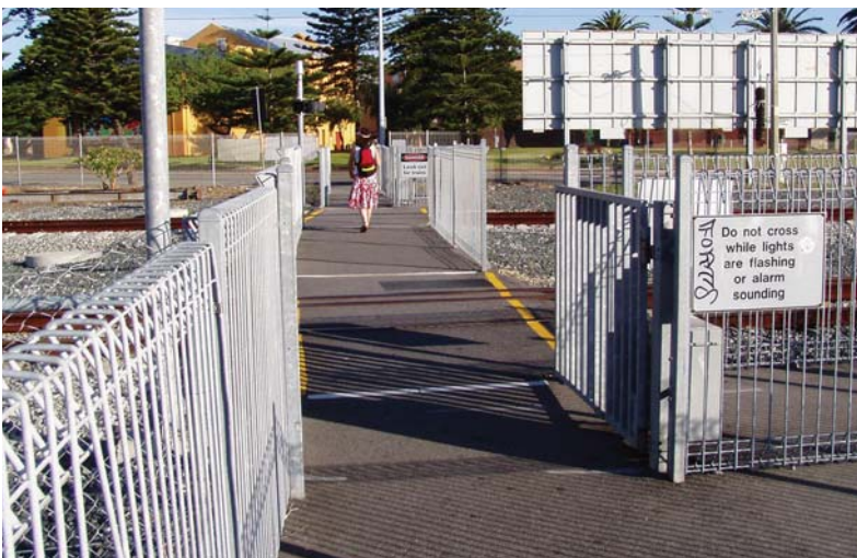
Photo 6.34 – Automatic pedestrian gates control double track crossing, Fremantle, Western Australia (Photo: Tim Hughes)
