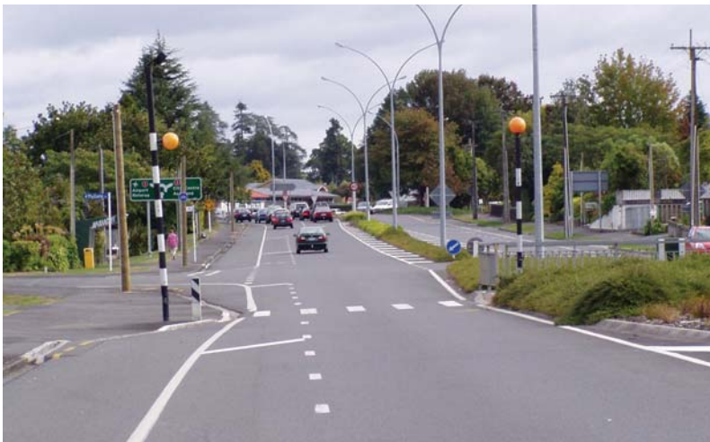
Photo 6.24 – Pedestrian zebra crossing, Hamilton (Photo: Tim Hughes)
