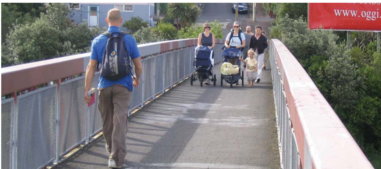
Photo 6.27 – Pedestrian overpass, Auckland (Photo: David Croft)
