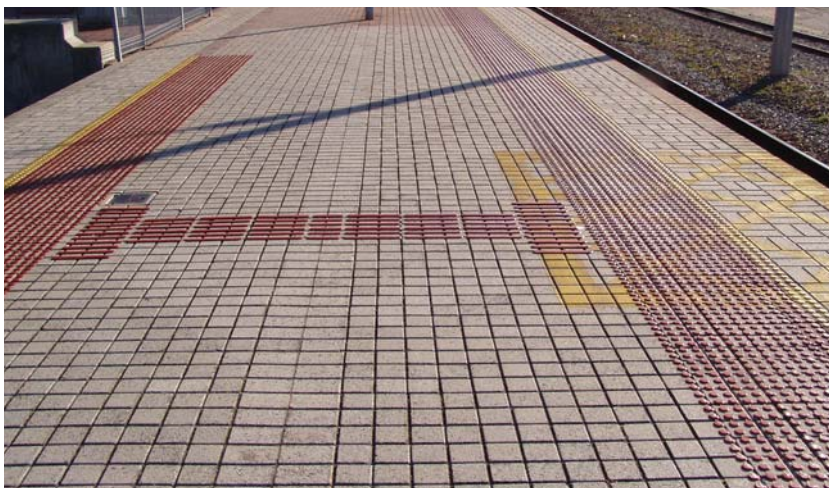
Photo 14.28 – Tactile paving treatment at railway station, Fremantle, Western Australia (Photo: Tim Hughes)
