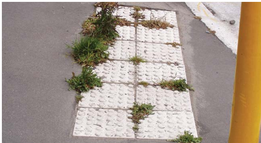
Photo 18.4 – Weeds growing around tactile paving (Photo: Tim Hughes)
