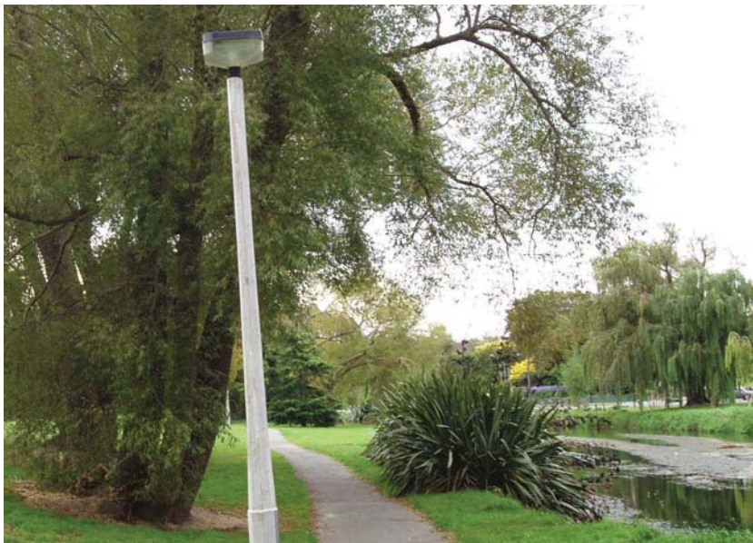
Photo 17.2 – Medium height lighting column, Christchurch
