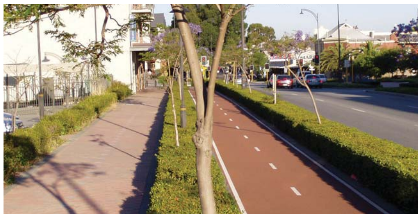
Photo 14.22 – Landscape barrier separates pedestrians and cyclists, Subiaco, Perth (Photo: Tim Hughes)
