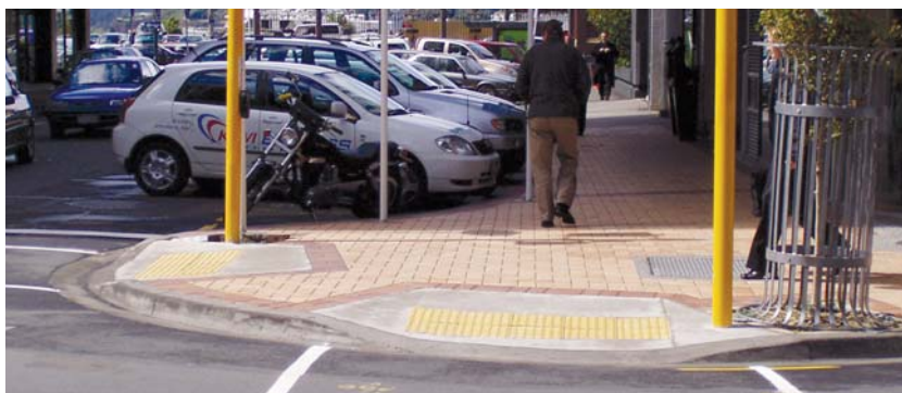
Photo 15.3 – Kerb ramp, Featherston St, Wellington (Photo: Tim Hughes)
