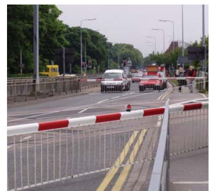
Photo 15.23 – Full automatic barriers, Hull, U.K. (Photo: Tim Hughes)
