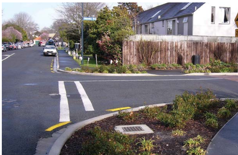
Photo 6.28 – Priority intersection, Christchurch (Photo: Andy Carr)
