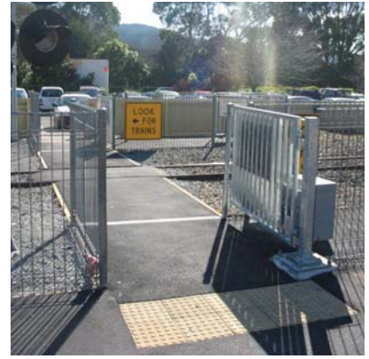
Photo 15.25 – Automatic pedestrian gate, Upper Hutt (Photo: Roy Percival)
