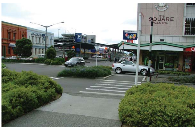
Photo 6.31 – Roundabout with zebra crossings on the approaches, Palmerston North CBD (Photo: Shane Turner)
