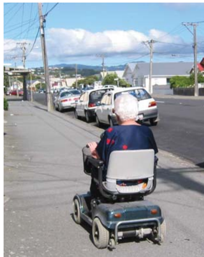
Photo 14.5 – Footpath with acceptable crossfall, Wellington (Photo: Lesley Regan)
