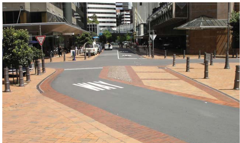
Photo 14.7 – Traffic calmed area with contrasting surfaces, Wellington (Photo: Shane Turner)
