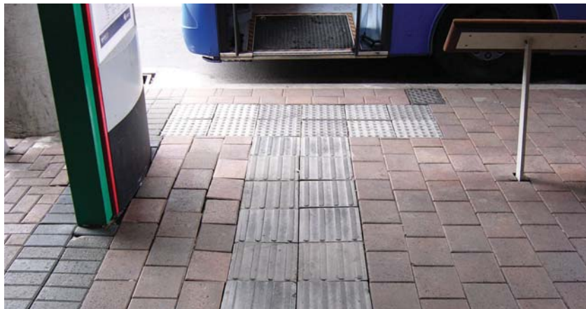
Photo 14.24 – Tactile paving at a boarding point, Christchurch (Photo: Paul Durdin)
