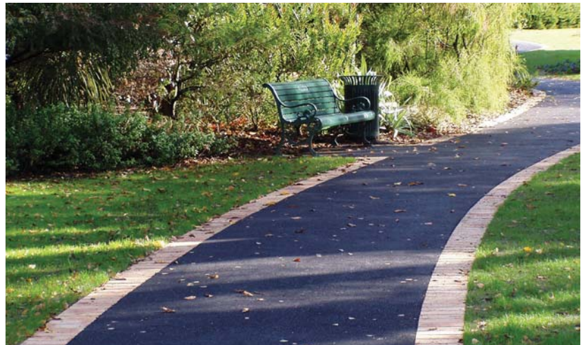
Photo 14.6 – Brick-lined asphalt path, Nelson (Photo: Tim Hughes)
