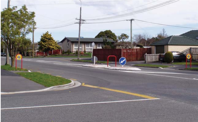
Photo 6.14 – Traffic island installed for safe routes to school, Christchurch (Photo: Tim Hughes)
