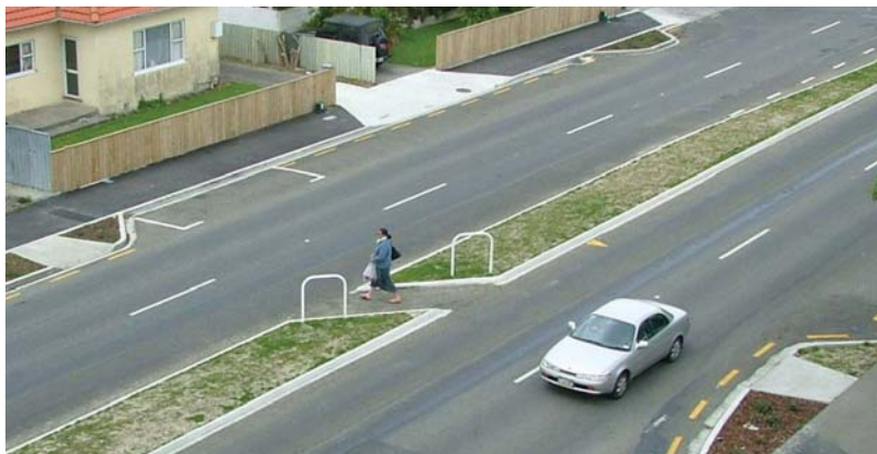
Photo 6.19 – Raised median with pedestrian cut-through, Palmerston North (Photo: Shane Turner) (note: tactile paving is missing)
