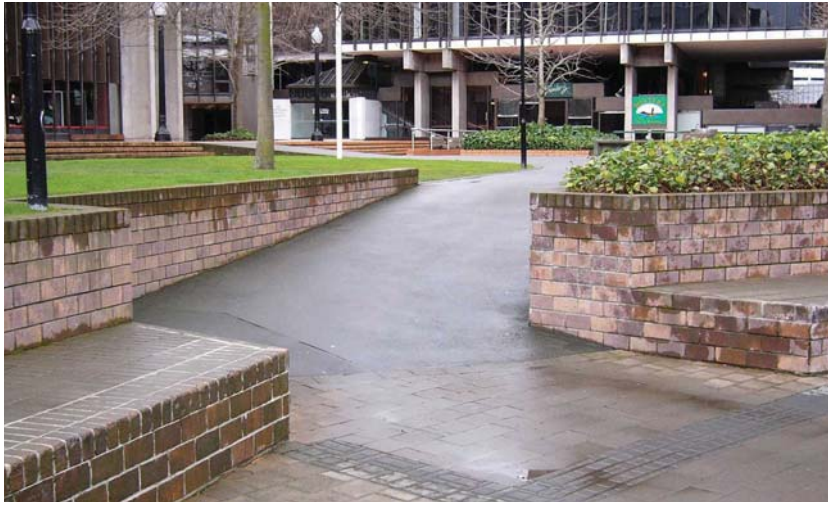
Photo 14.4 – Gradient in footpath between two levels, Christchurch (Photo: Andy Carr)
