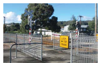
Photo 15.24 – Pedestrian rail crossing maze, Upper Hutt (Photo: Roy Percival)
