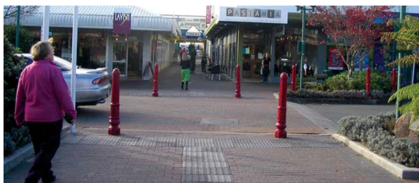
Photo 15.5 – Blended kerb crossing at platform, Taupo (Photo: Else Tutert)
