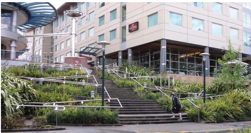
Photo 6.6 – Steps and zig-zag ramp, Hamilton (Photo: Shane Turner)
