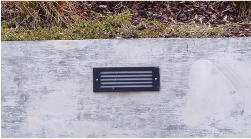
Photo 17.1 – Low mounted lighting in wall by ramp, Queenstown (Photo: Tim Hughes)
