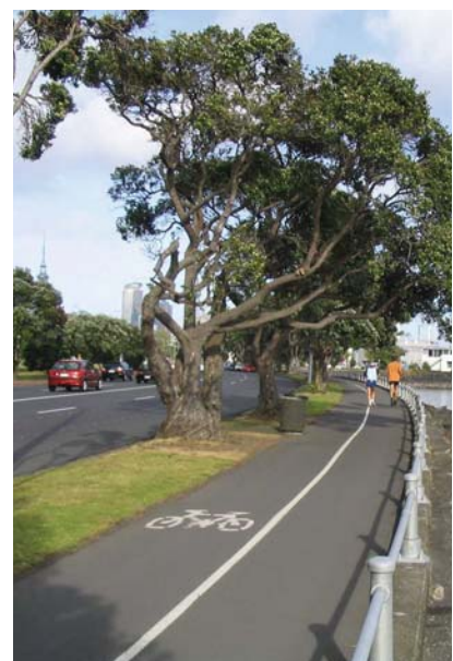
Photo 6.9 – Segregated path, Auckland (but substandard width)
