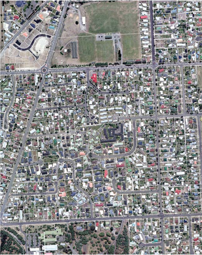
Figure 4.1 – Externally distributed network with poor internal connections apart from some narrow paths, Blenheim (Source: Grant Crosswell, Marlborough District Council)
