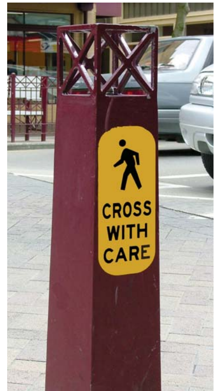
Photo 15.10 – Sign on bollard delineates edge of roadway, Palmerston North (Photo: Tim Hughes)
