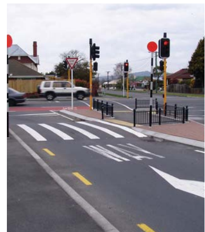
Photo 15.17 – Platform pedestrian crossing free turn, Northlands mall exit, Christchurch (Photo: Tim Hughes)
