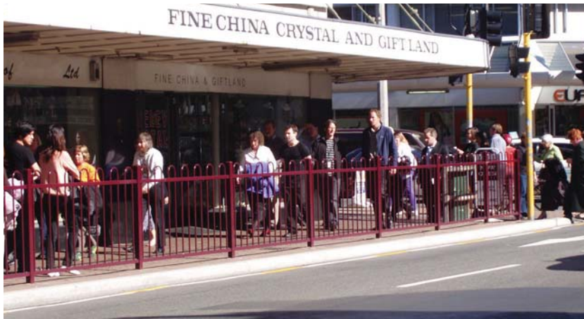
Photo 16.7 – Pedestrian fence, Christchurch
