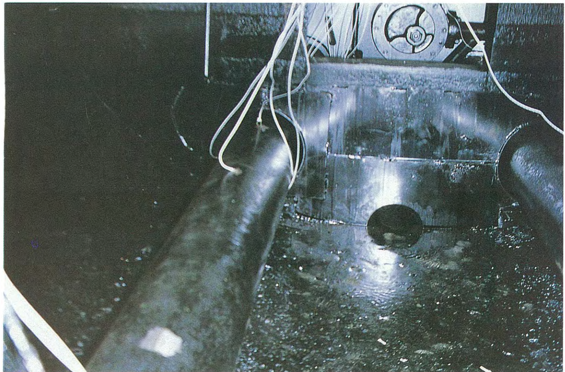
Thermocouple probes welded to flame tube inside tank.
