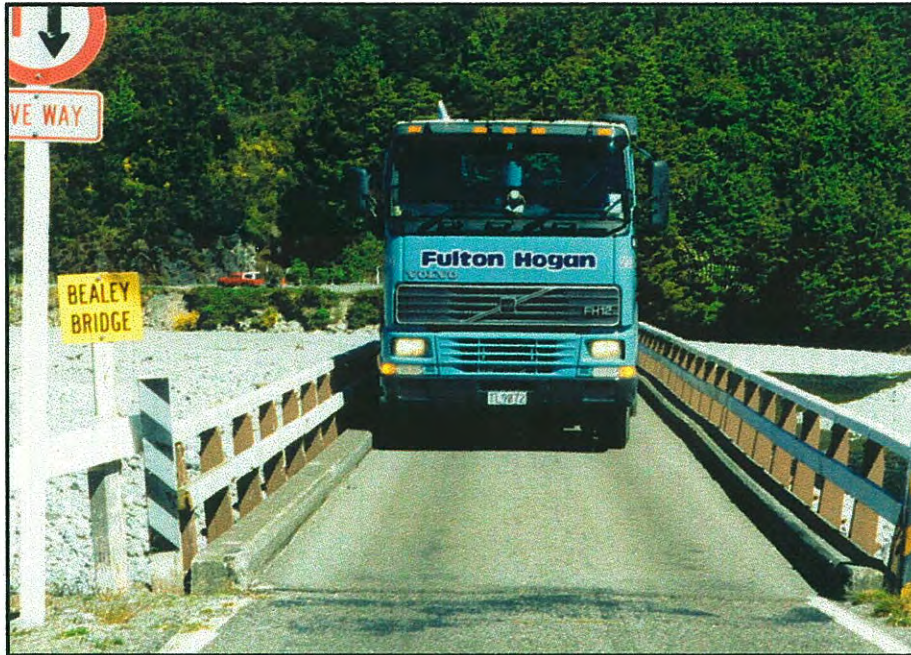
Figure 4.6 Known vehicle on the bridge during testing.
