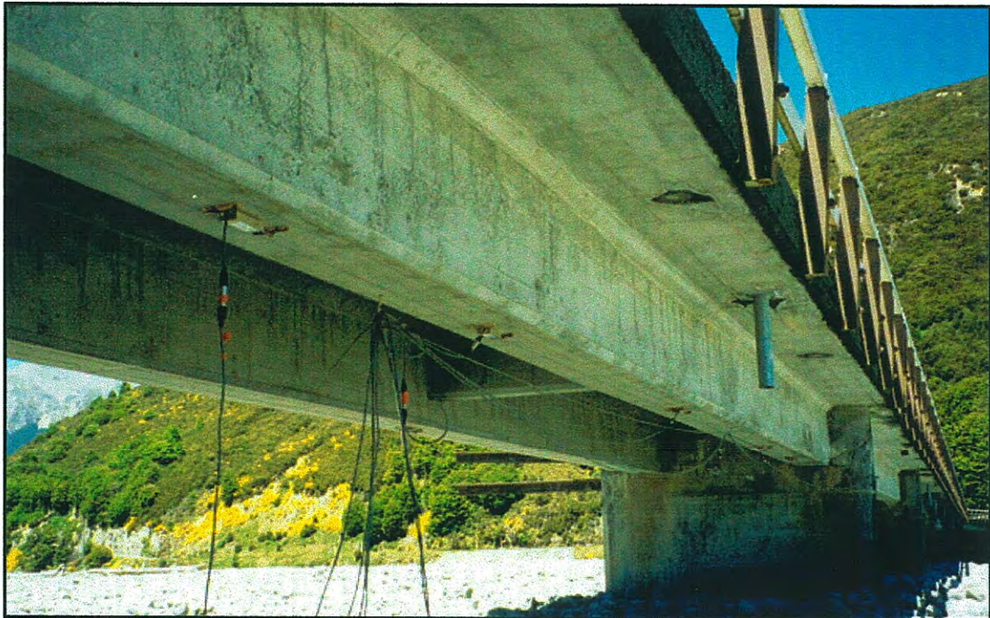
Figure 4.2 Instrumentation on Girder 1, Span 2.
