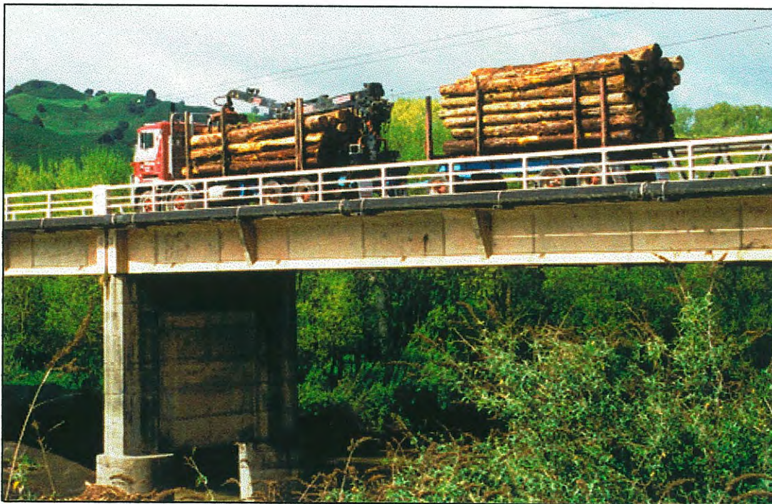
Figure 4.6 The known vehicle on the bridge during the testing.
