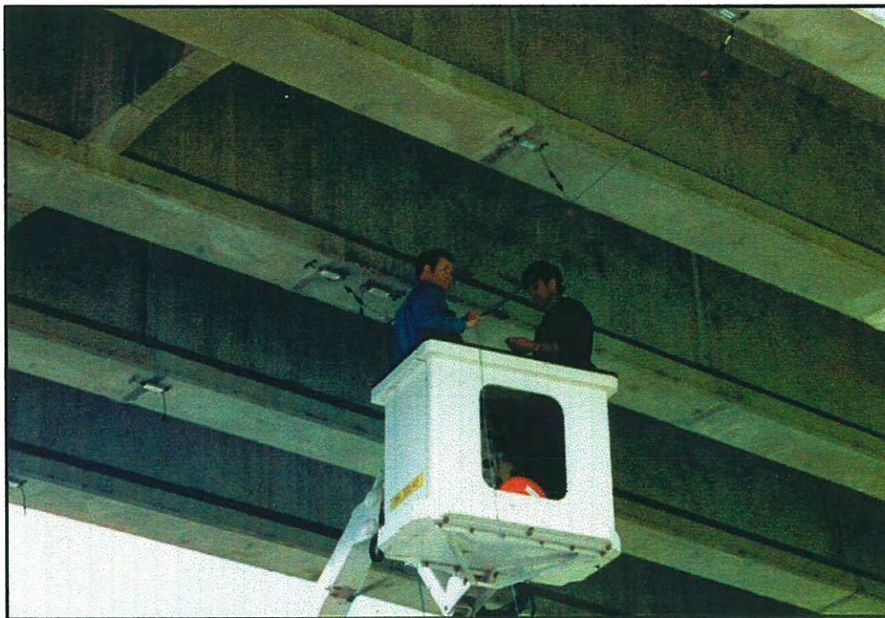
Figure 4.3 Installation of instrumentation on girders of the Wanganui Bridge.
