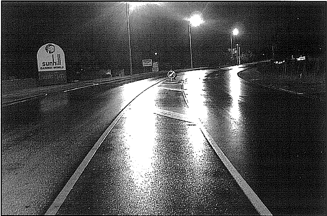
Figure 6.1 Standard pedestrian refuge island at night.
