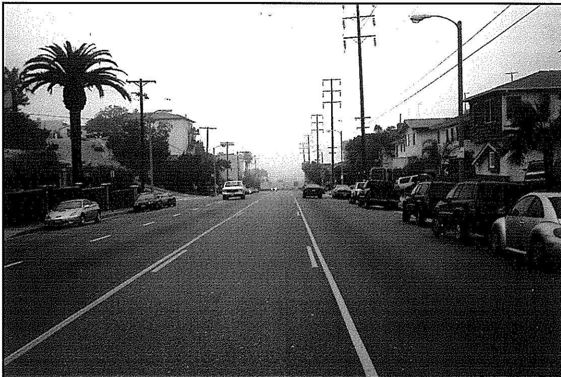
Figure 2.3 Two-way left-turn lane, as used in the US, with two sets of lane-line markings, bordered by two yellow lines.
