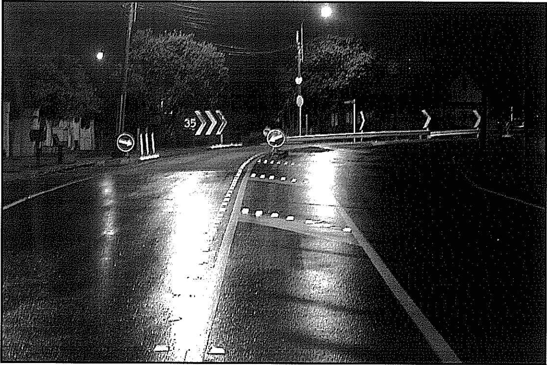
Figure F1 Pedestrian refuge island with no-overtaking line and rrpms on approaches, at night.
