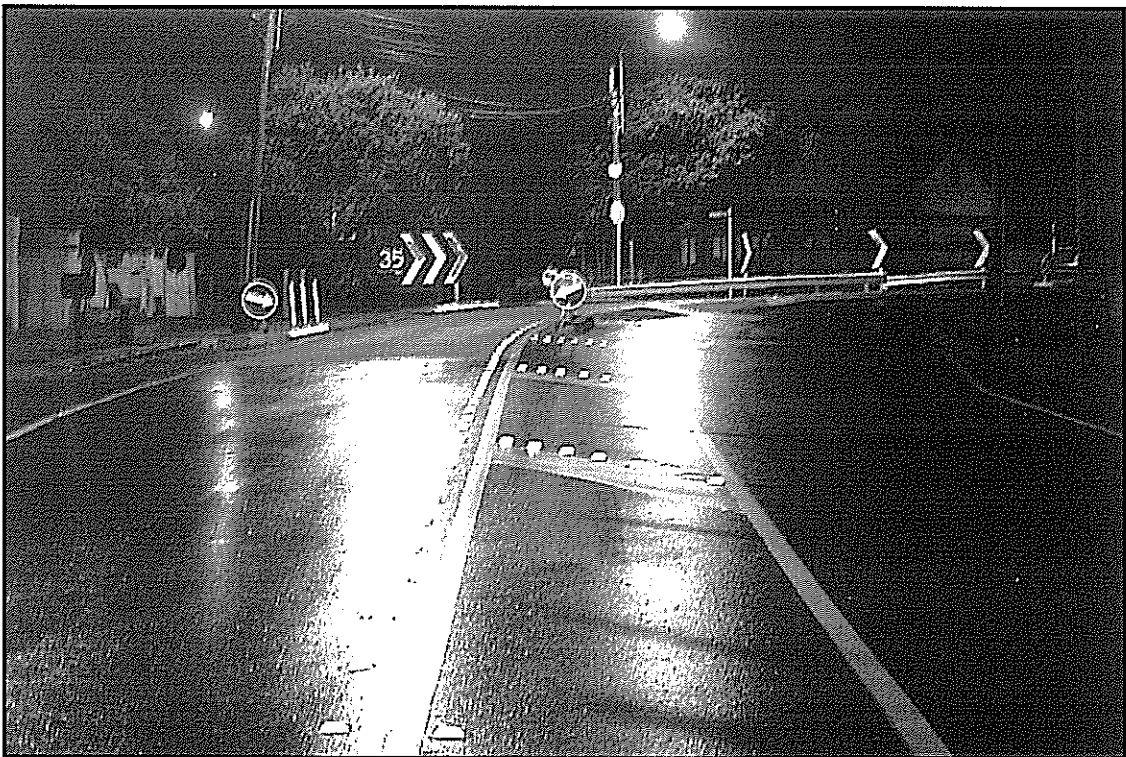
Figure 6.2 Pedestrian refuge island with no-overtaking line and rrpms on approaches, at night.
