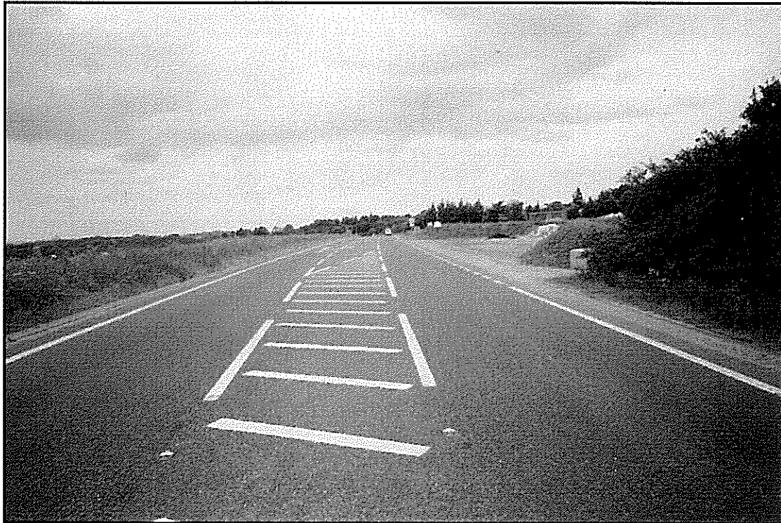
Figure 2.2 Ghost island, as used in the UK, with dashed edge line to separate traffic flows.
