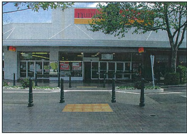
Pedestrian lines removed
