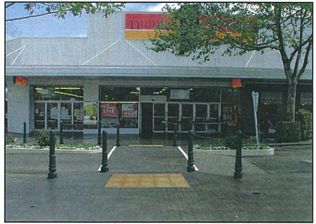
Driver lines removed
