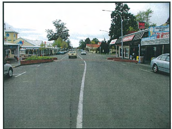
Figure 2.3 Driver's view of a paved traffic-calming speed hump.
