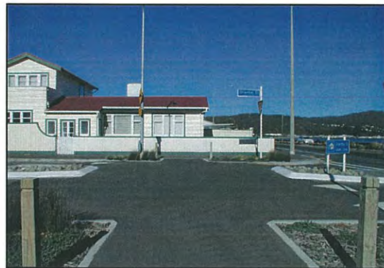
Figure 4.5 Pedestrian–vehicle space with tactile surfaces removed.
