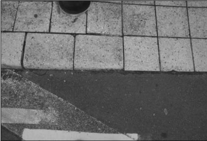
Figure C26 Close-up view of accident site 13
