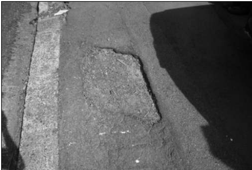
Figure B28 Close-up view of accident site 14
