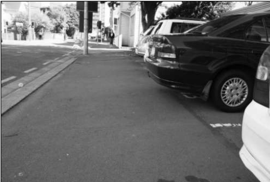
Figure B13 Long-shot view of accident site 7
