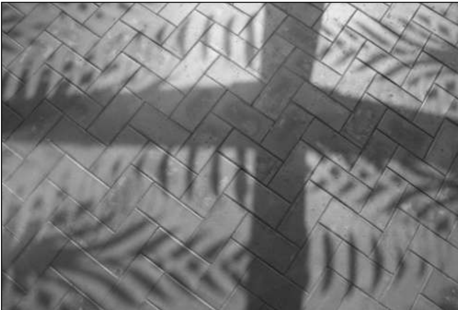
Figure B16 Close-up view of accident site 8
