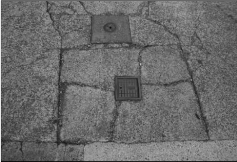
Figure B18 Close-up view of accident site 9
