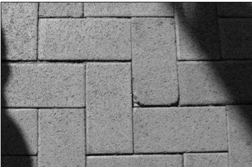
Figure B24 Close-up view of accident site 12
