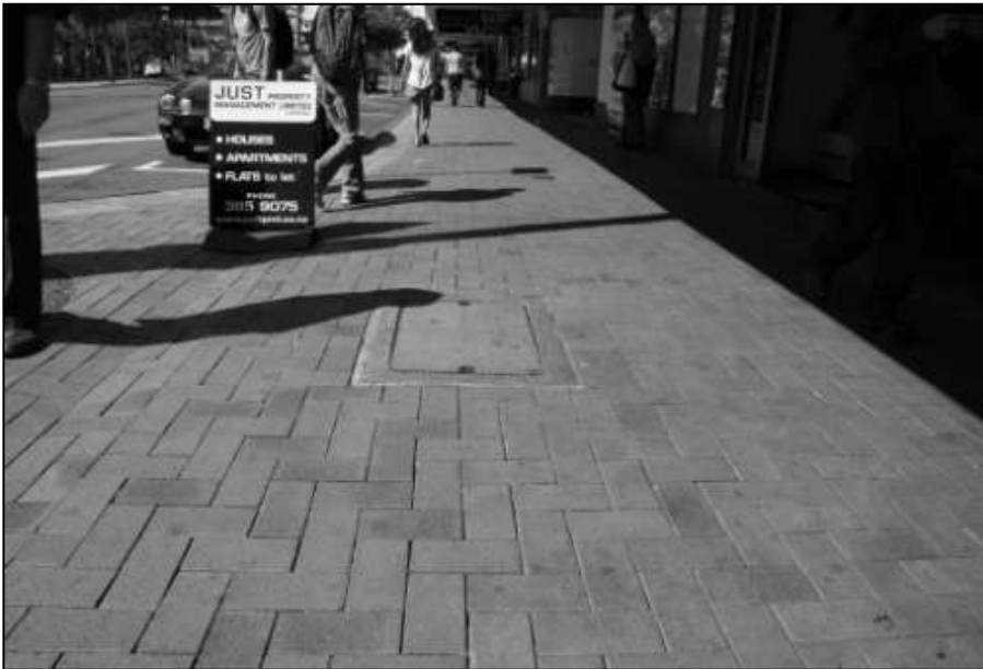
Figure B23 Long-shot view of accident site 12
