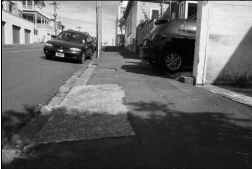
Figure B27 Long-shot view of accident site 14
