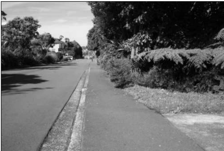
Figure B9 Long-shot view of accident site 5
