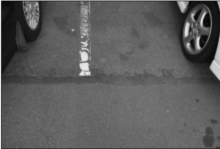
Figure B14 Close-up view of accident site 7
