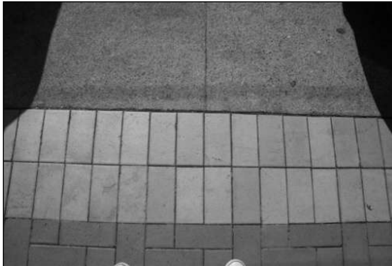
Figure B22 Close-up view of accident site 11
