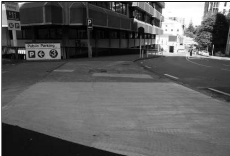
Figure B17 Long-shot view of accident site 9
