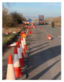
The TTM involved three permanent lane closures to increase the working area. HRS Intellicone Smart Taper was used as an enhanced safety measure. This provides immediate digital notification of any strike. The metric for determining success was time to reinstatement compared to time to reinstatement without the smart cones.
