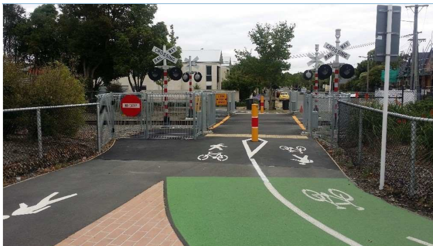
Figure 5-2: Transition between shared path, footpath and separated cycleway, Matai Street, Christchurch
