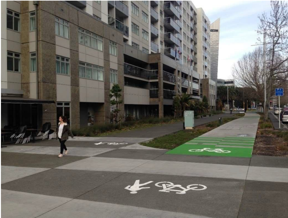
Figure 5-3: Transition between shared path, footpath (note: missing recommended pedestrian symbol at start of footpath) and separated cycleway, Beach Rd, Auckland
