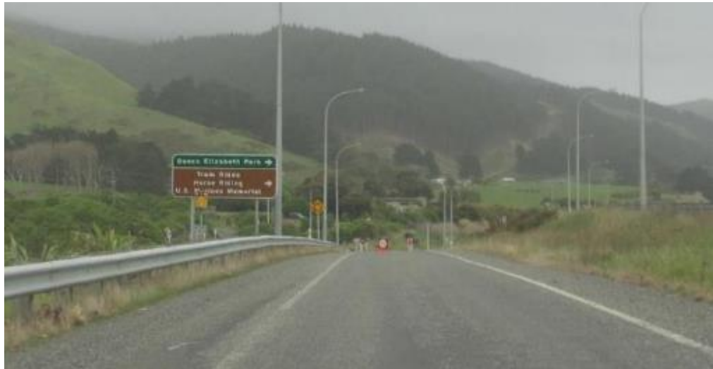
Figure 10: Poor forward view to roundabout at the end of the southbound off-ramp
