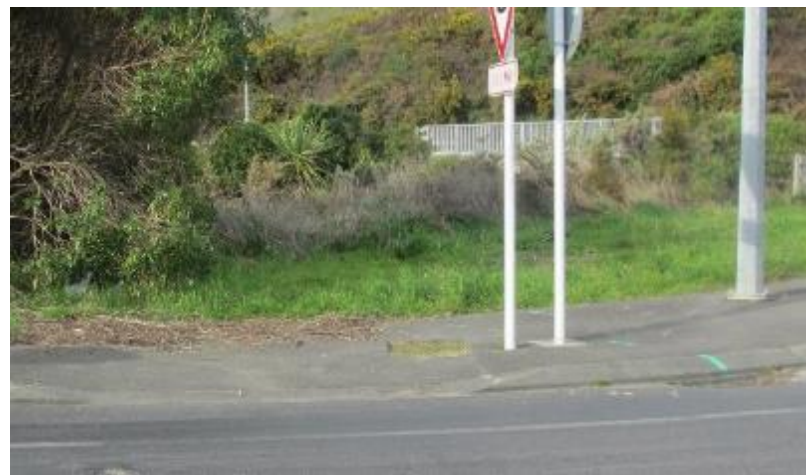
Figure 7: Signs and streetlight obstructing the path on the eastern side of the southbound off-ramp
